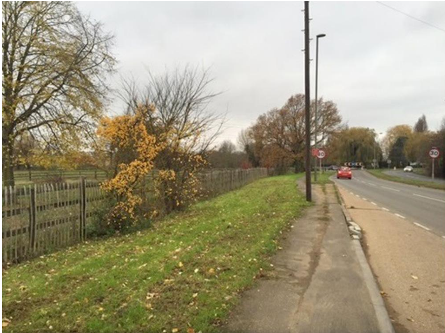
Figure 1 : View of the application site to the south west with the A308 to the north west
